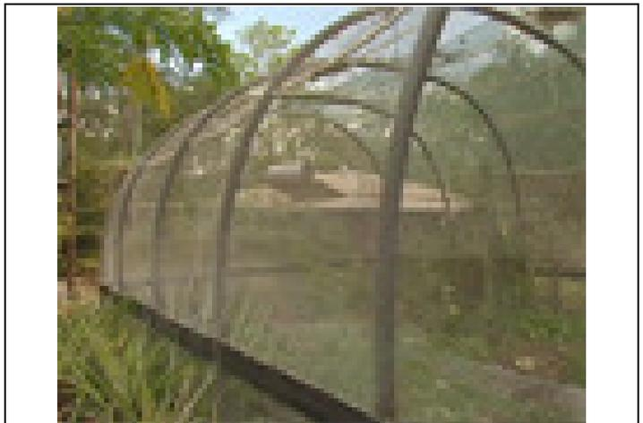
Temporary structure made of heavy duty ag pipe and shaded cloth which could be adapted as a cover for feeders and waterers
